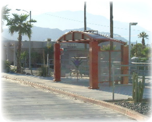
This shelter located in Palm Springs, California allows air to circulate. The panels are constructed of perforated metal to allow airflow while maintaining good visibility of the surrounding area.
