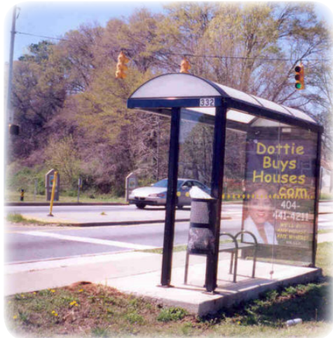
The bus shelter is placed on a concrete block that is level with the sidewalk. It provides a stable surface for wheelchair users and does not impose on the bus landing pad area. Photo taken in Mableton, Georgia.
