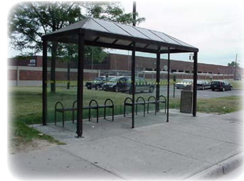
This shelter in Rochester, New York, provides two openings for entering and exiting, as well as wind protection from the northern climate.
