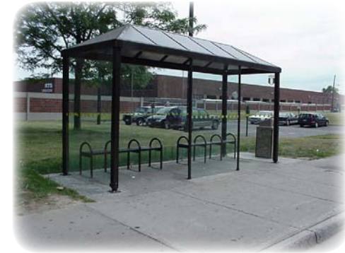
This shelter in Rochester, New York, provides two openings for entering and exiting, as well as wind protection from the northern climate.
