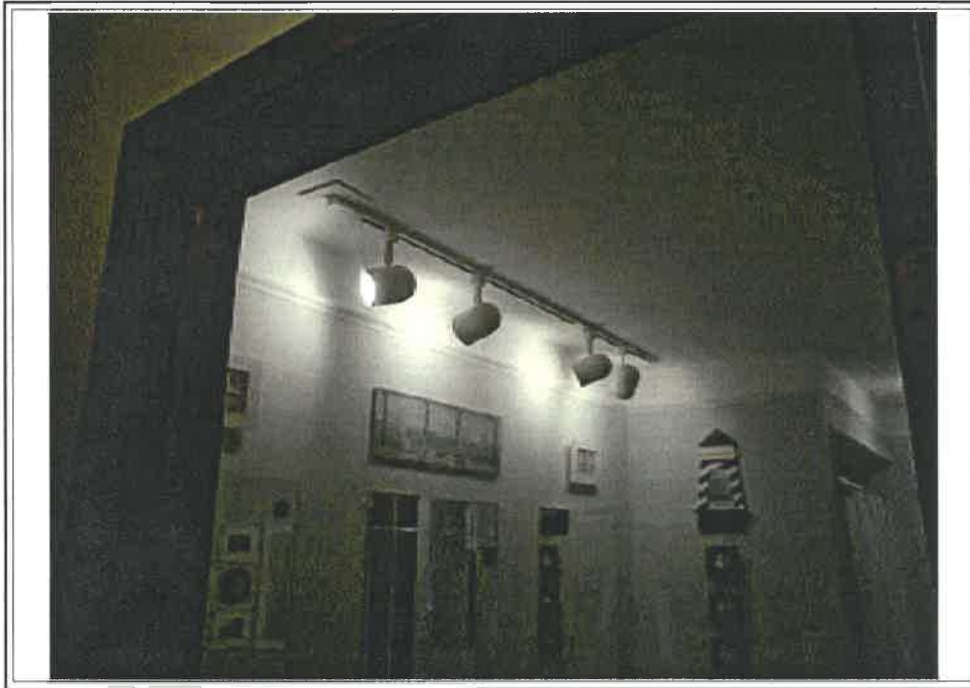
Track lighting above double vanity with three mirrors in hall bath shown in preceding photo.
