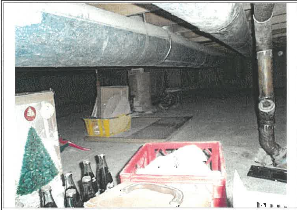
View of crawl space
