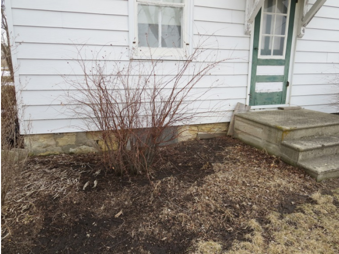
Photograph 3 Detail showing limestone foundation at west facade.
