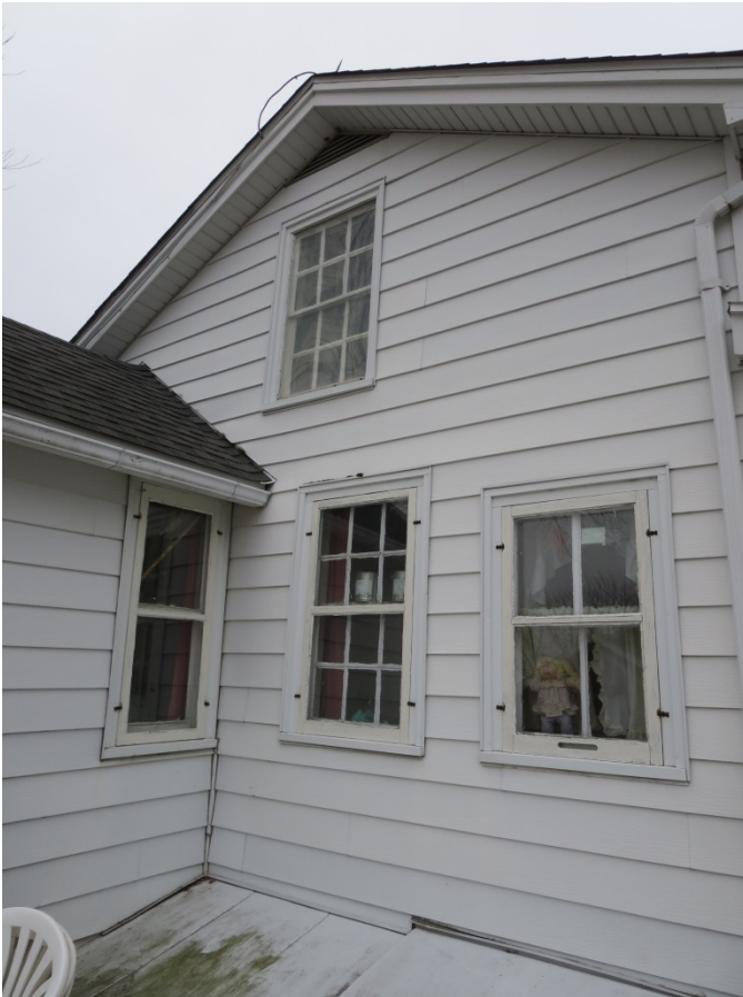
Photograph 10 Detail of rear (east) facade showing various historic window configurations.
