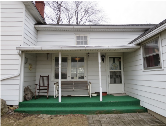
Photograph 18 Detail of side (south) porch.
