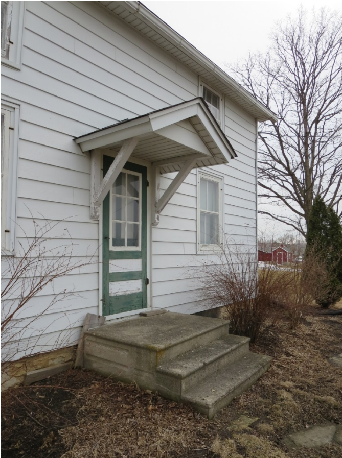
Photograph 2 Detail of west entrance.
