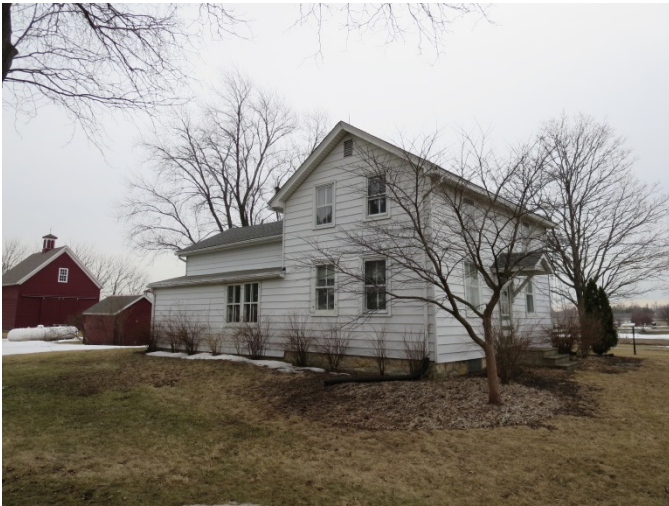
Photograph 5 Three quarter view showing north and west facades.
