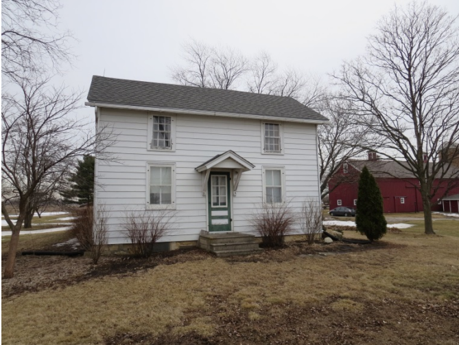
Photograph 1 Front (West) Facade.
