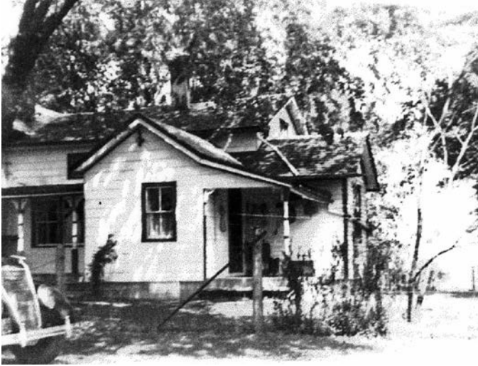
Photograph 10 Southeast corner of house showing open porch at rear, 1940.
