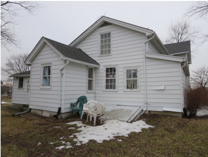
Photograph 8 Rear (East) Facade.
