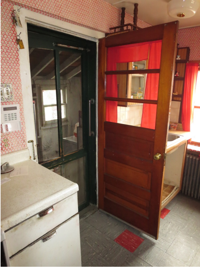
Photograph 15 Interior view of rear door. This main entry door appears to be from a date later than the selected restoration period. The screen door here is historic, but may have been located at a different opening.
