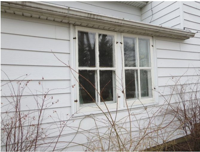
Photograph 7 Detail of first floor windows at north facade.
