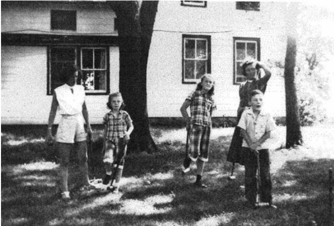
Photograph 11 North Facade, 1954. Note window openings at attic story of rear wing.
