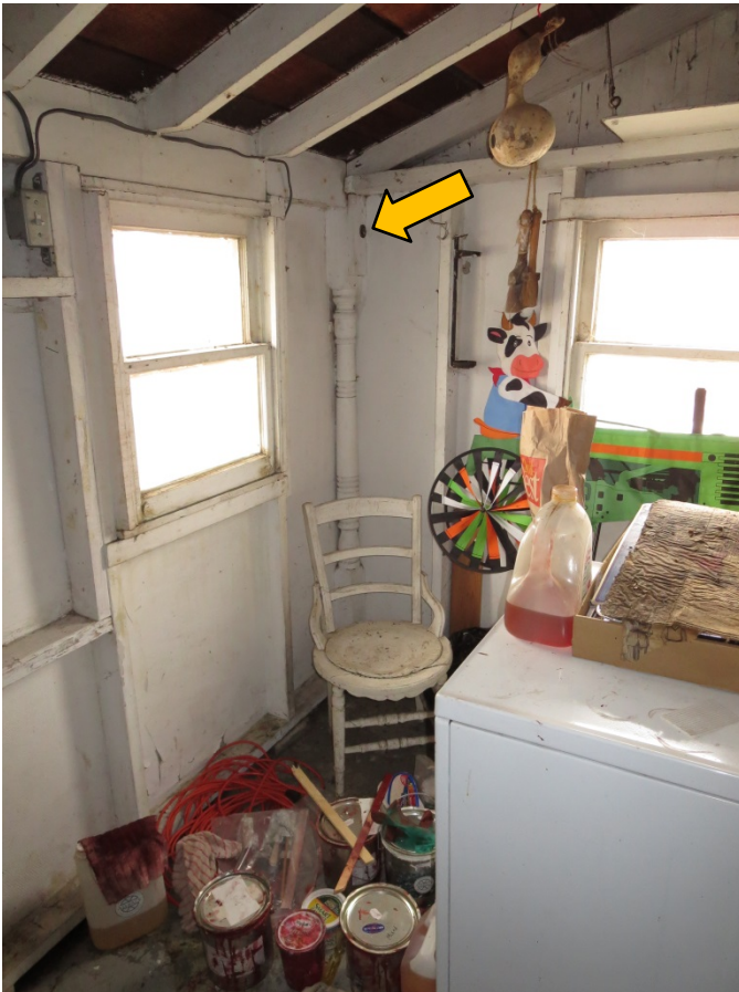
Photograph 12 Interior view of enclosed porch showing historic wood corner post.
