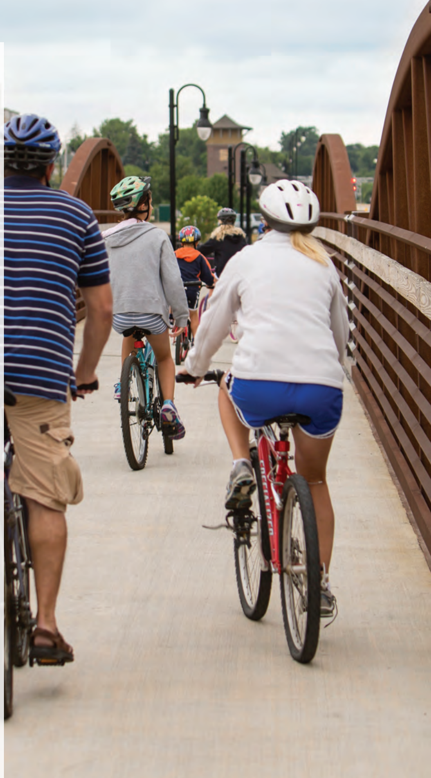
Pedestrian Bridge providing pedestrian access across LaGrange Road.
