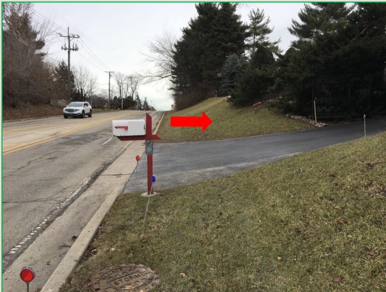
Existing embankment area (looking east)
