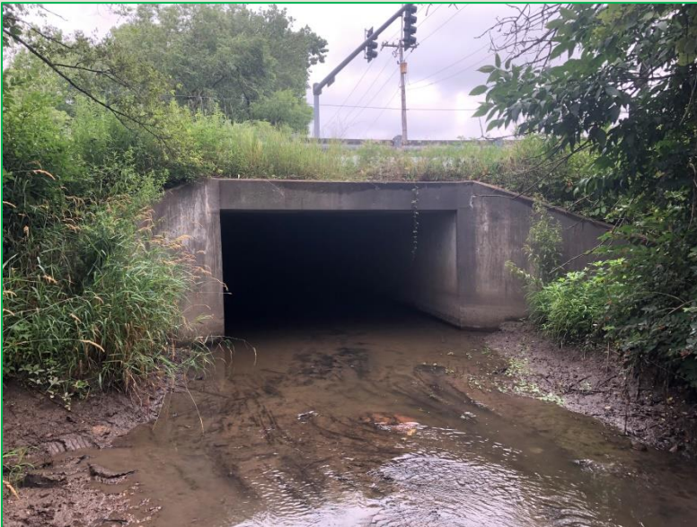
167 th Street at Wolf Road (SW corner – existing culvert)
