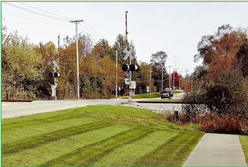
Existing RR Crossing (167 th Street – looking east)
