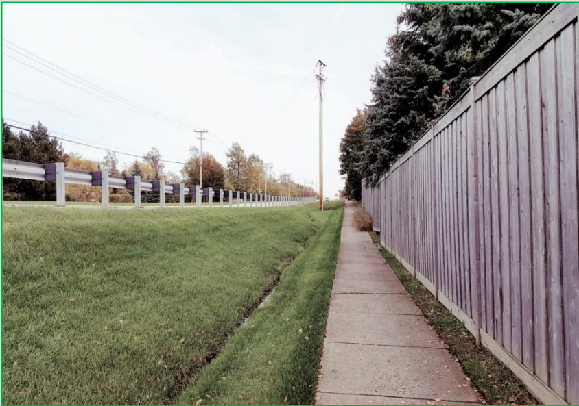
Existing embankment area (looking east)
