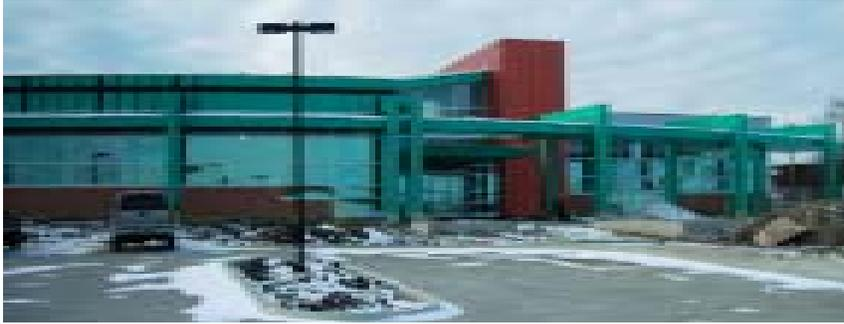
The Orland Park Police Facility, at 151st Street and Ravinia Avenue, will be substantially completed in mid-February. The green covering on the outside of the building is not the final facade. This is the water proofing material.
